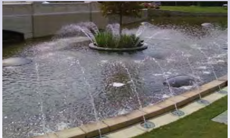
Liner "whale backs" can result from accumulated ground water, air bubbles or a combination of the two. This occurs when there is no venting or drainage installed below the liner.
